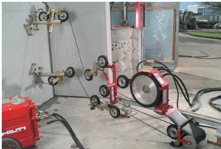
Fig. 16 Portable wire machine making a vertical cut in a concrete wall (Courtesy of Hilti Corp).
